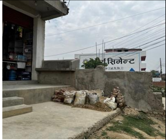
Corner of the boundary wall likely to be affected
