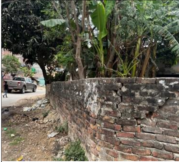
Likely affected boundary walls
